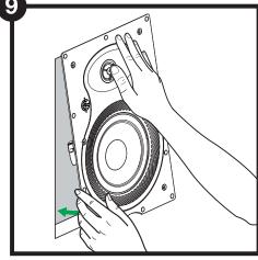
Insert the speaker into the wall and ensure that it is properly seated.
